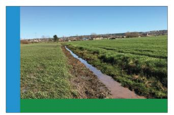
**Two-Stage Ditch - "**The Two-Stage ditch requires less maintenance. The one-stage ditch fills in with silt and sediment quicker and requires more maintenance. It's good to keep the ditch's slopes covered in vegetation to prevent erosion."
